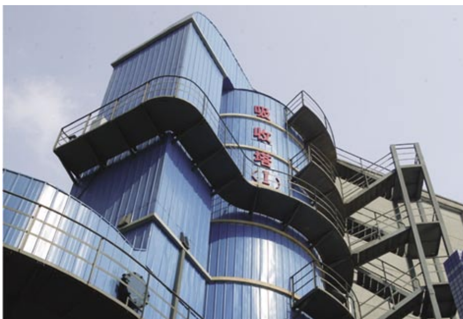
Sulphur dioxide absorber tower, Huasheng Project in Hubei Province
